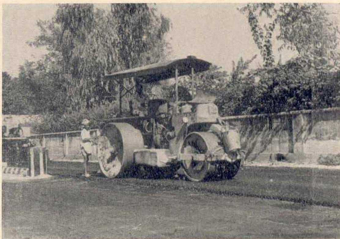
Photo 2. 3-Wheel Steel-tyred roller
